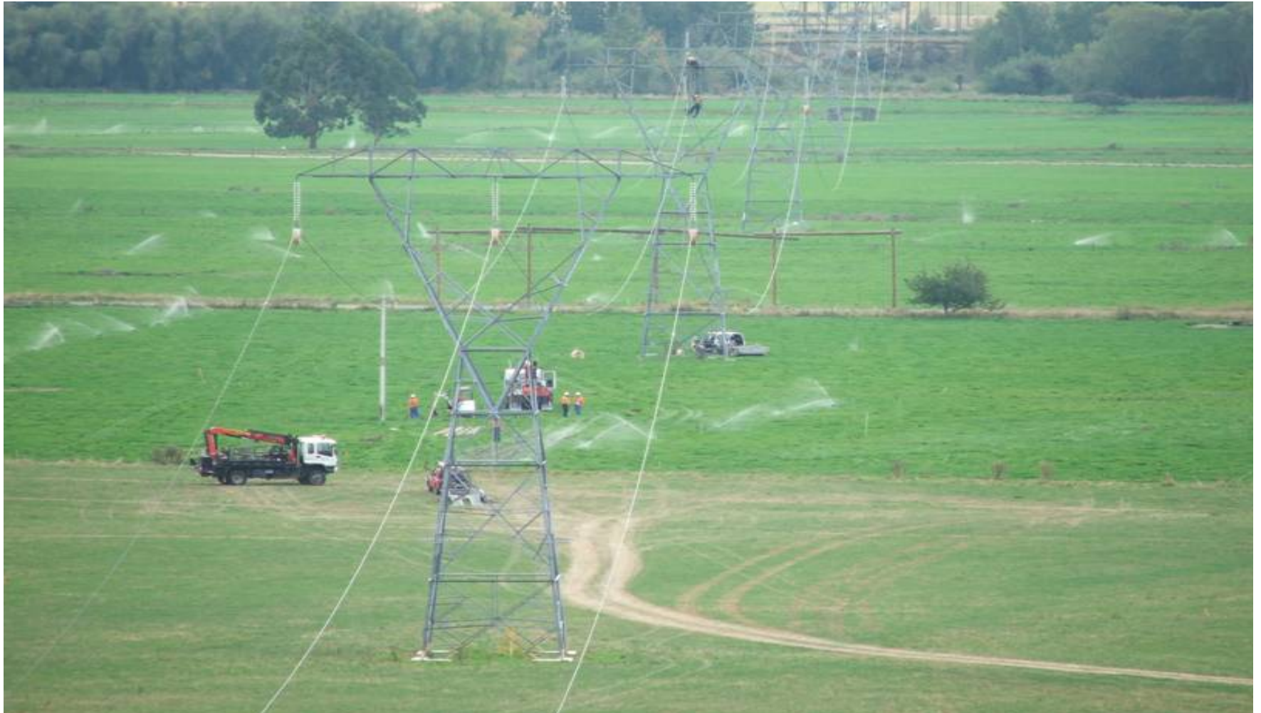
Roxburgh-Livingstone, wiring crews in action
