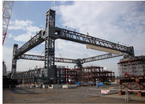
Provisional Assembly of Framework for Protective Cover
